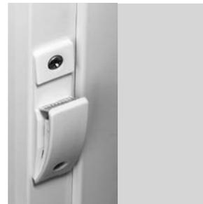
The weather sensor is mounted on the outside of the window. This detects rain and snow as well as the temperature and wind force at the window, and it closes the window if necessary. Unfortunately, this sensor was not used in this project.
